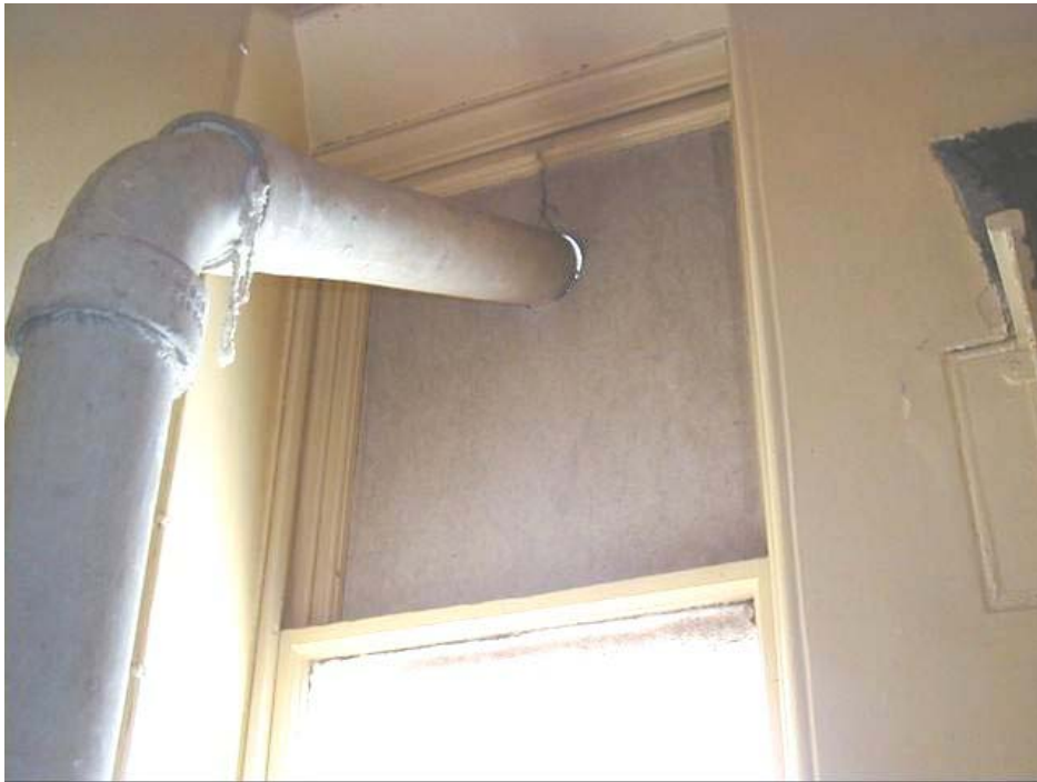
Figure 4.5 Asbestos cement flue with asbestos rope seals passing through asbestos infill panel.
