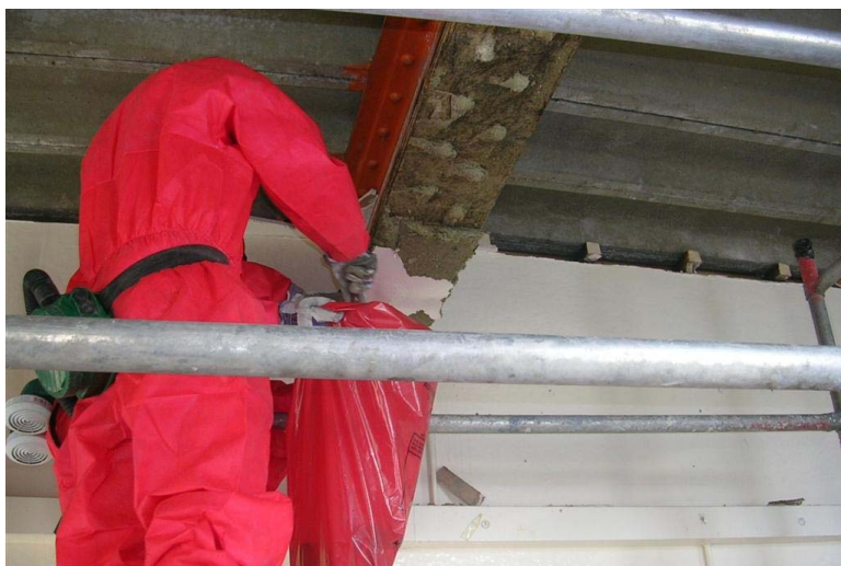
Figure 12.11 Bagging waste close to the point of removal to prevent spread and minimise exposure.
