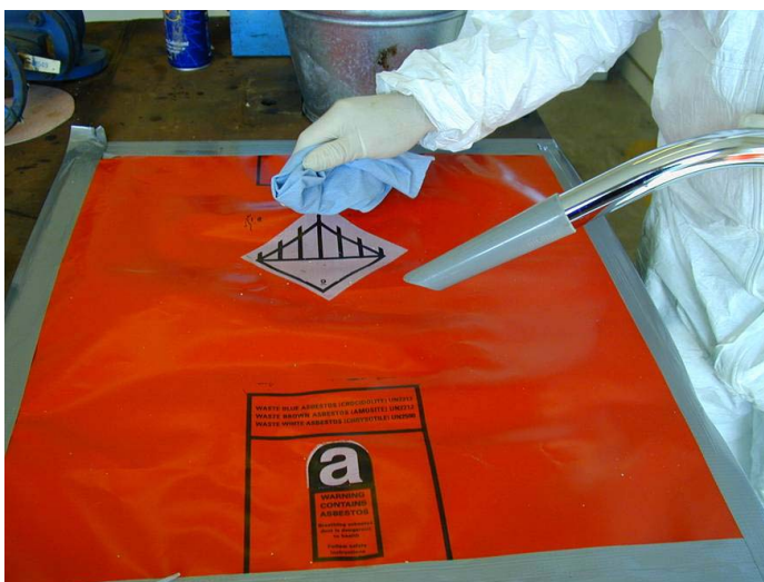
Figure 11.7 Cleaning up the work area carefully, with H-Type vacuum cleaner and wet waste rags.
