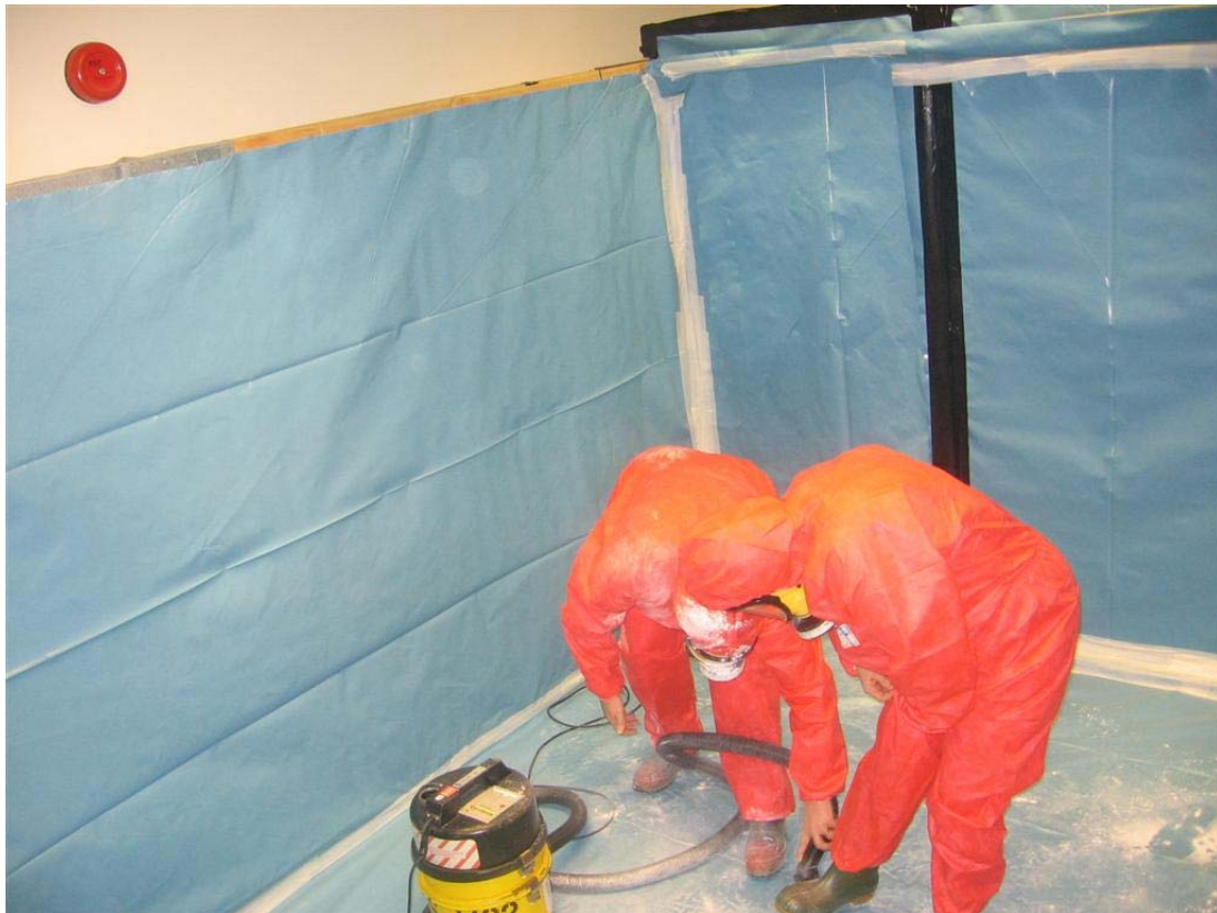
Figure 7.1 Practical training in the use of Type-H vacuum cleaners to remove simulated contamination (talcum powder). Figure provided by the UK HSE.
