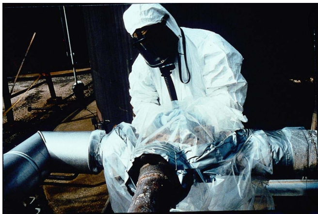
Figure 12.12 Glovebags used for controlled removal of asbestos lagging (photographs provided courtesy of INRS; copyright INRS)
