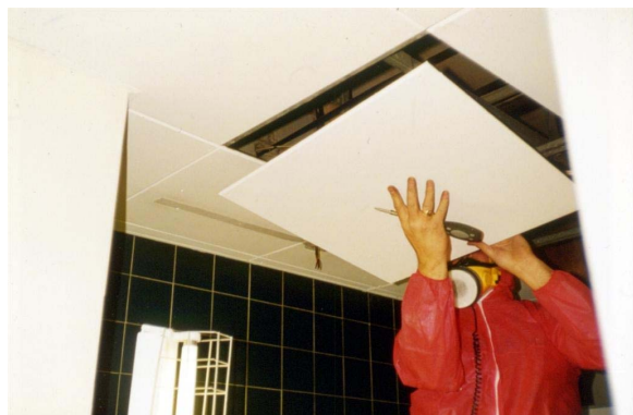
Figure 12.13 Careful removal of an asbestos tile
