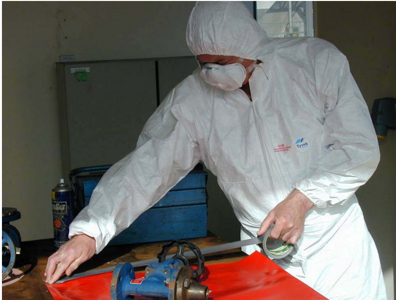
Figure 11.3 Use of tape and polythene sheeting to protect a work area before cleaning asbestos gaskets from a valve
