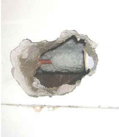
Figure 4.4. Penetration of a wall to show asbestos pipe insulation.
